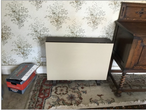
Photo - 91 Storage heater in front reception
