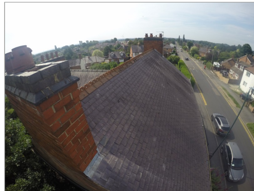
Photo - 6 Roof line
