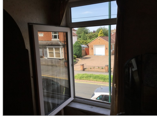
Photo - 29 Front bedroom window
