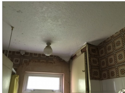
Photo - 46 Bathroom ceiling
