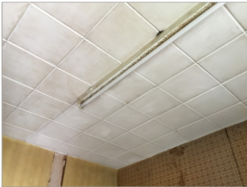
Photo - 43 Polystyrene tiles
