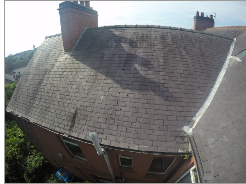
Photo - 8 Left elevation of rear projection
