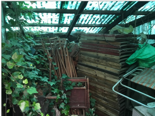
Photo - 102 Timber framed storage area off rear of outbuilding
