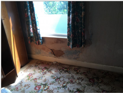
Photo - 62 Rear wall in middle bedroom
