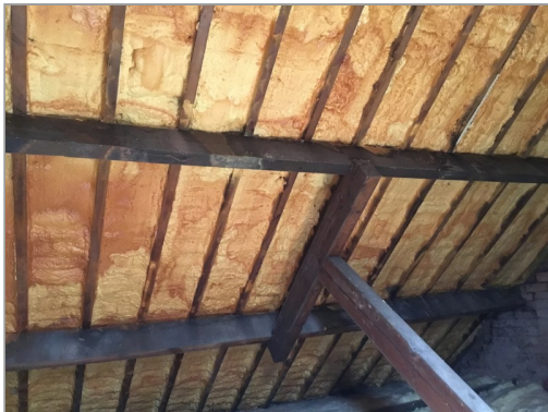
Photo - 37 Foam applied to underside of slates.
