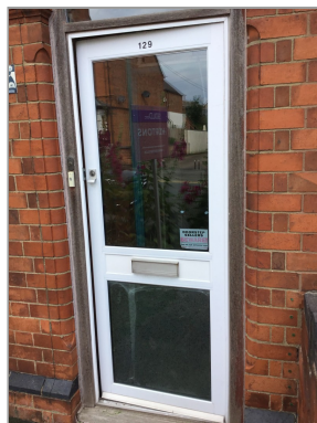
Photo - 30 Front door
