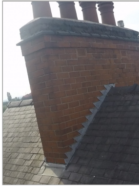
Photo - 3 Front elevation of rear chimney
