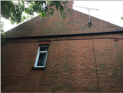
Photo - 18 Left gable
