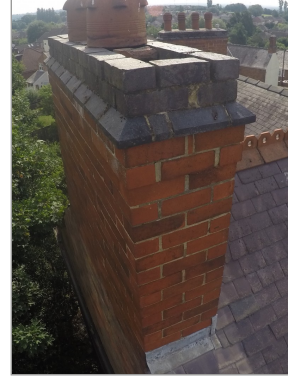
Photo - 2 Front chimney
