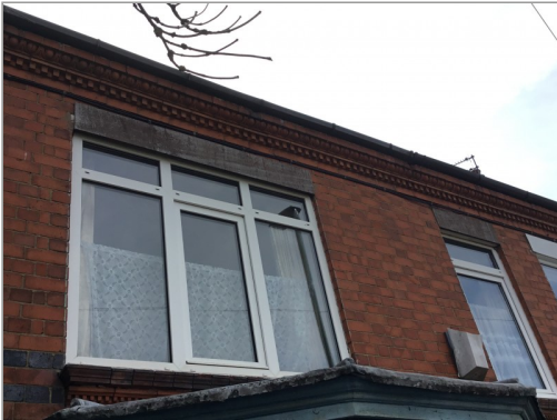
Photo - 14 Timber cladding over lintels to front elevation
