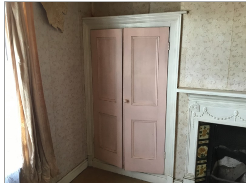
Photo - 78 Front bedroom
